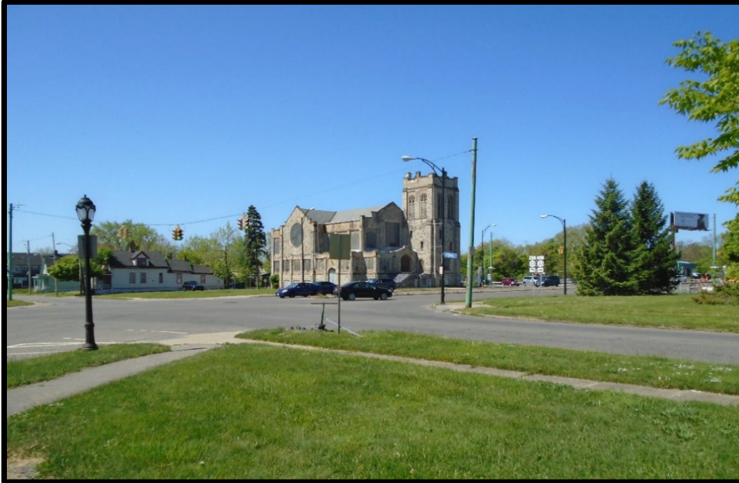
View looking southwest from Best Street and West Parade Avenue which is also the West Parade Circle entrance to Martin Luther King Jr. Park.
