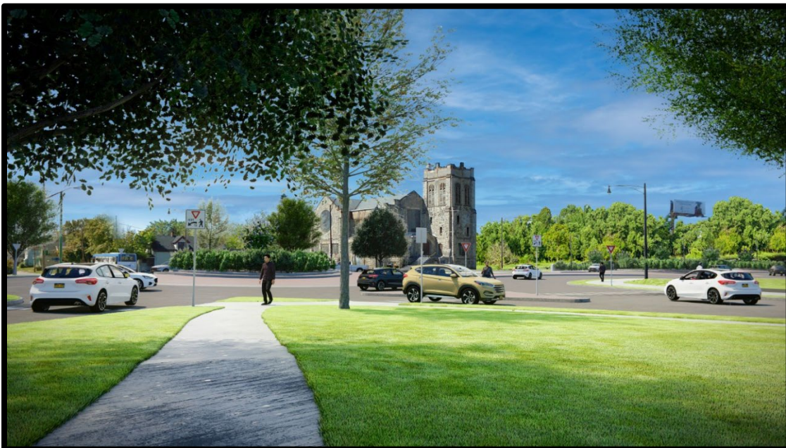
Note: This simulation is a representation of the Build Alternative in the preliminary design phase. Project elements shown may be updated during final design.
