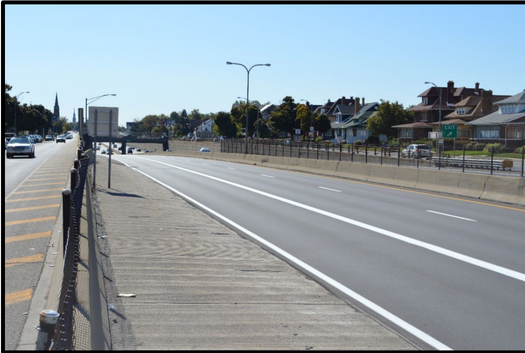
View looking south from the shoulder of the Kensington Expressway eastbound toward the proposed north tunnel portal.
